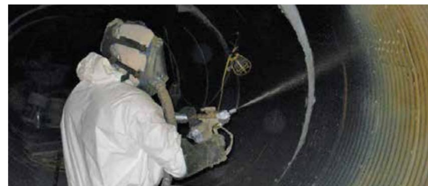
Polymeric SAPL being applied to an asset. Image courtesy of Sprayroq.
