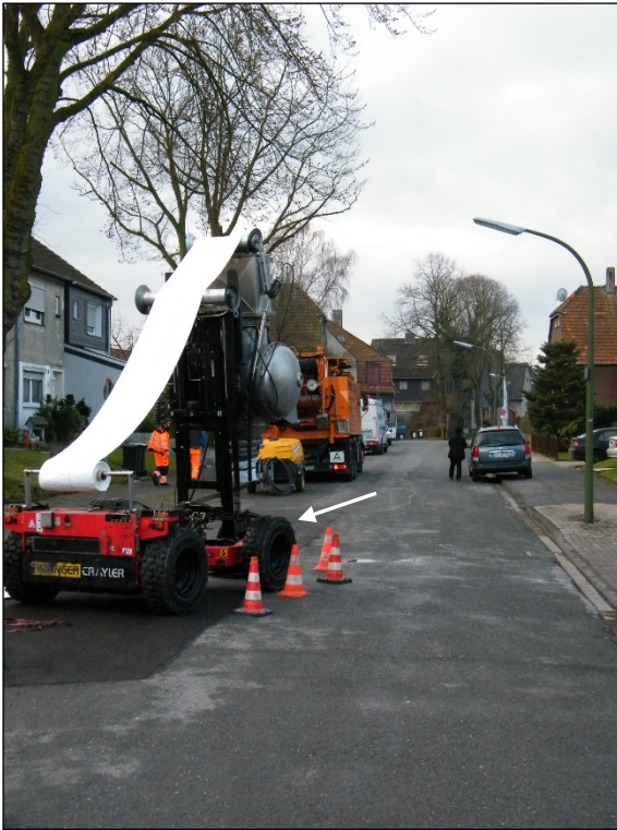
Figure B12. Inversion Manhole (3823) Looking Towards Termination Manhole
