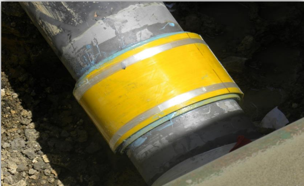
Figure 3.6. Repair Method for Corroded Joint
