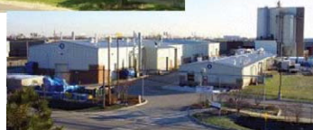
Energy & Environmental Technology Center
