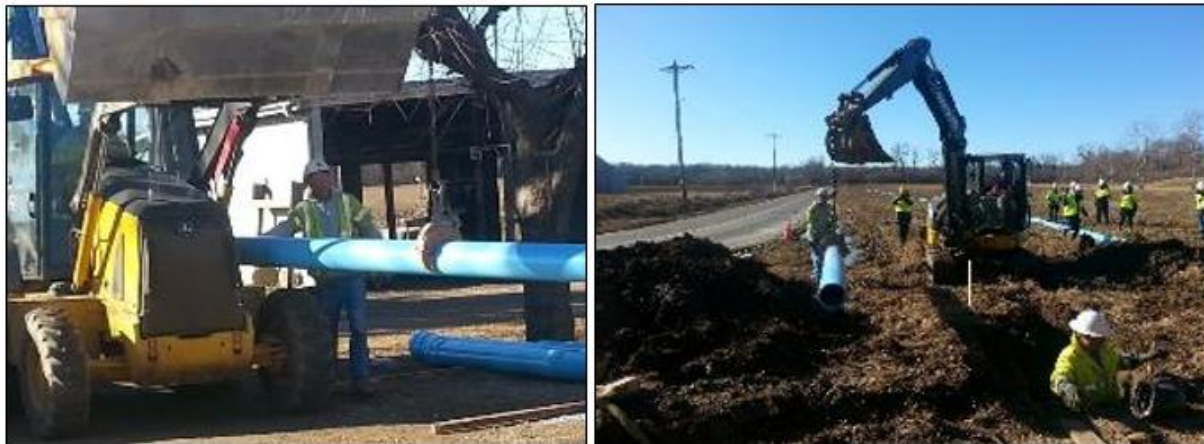
Figure 5.4 iPVC delivered to the trench
