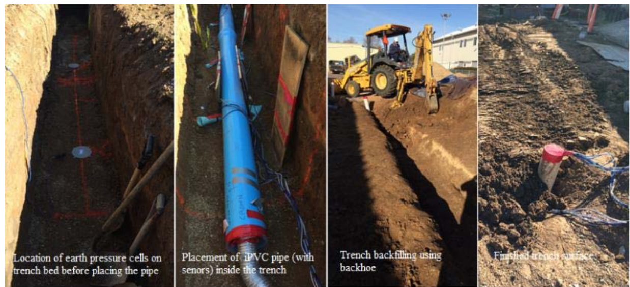
Figure 3.26 Pipe and sensor installation (Test 2)
