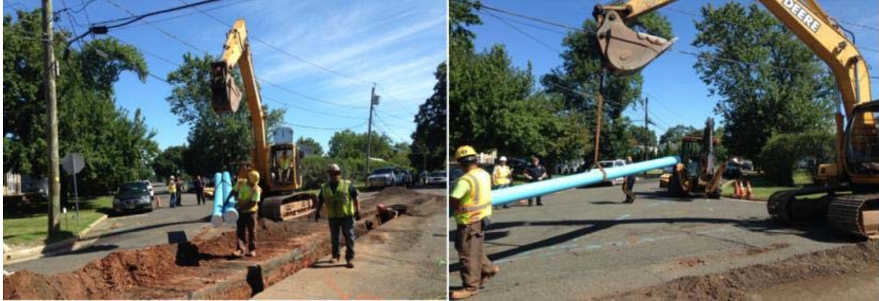
Figure 5.8 Contractor installing new iPVC pipe at Manville, NJ
