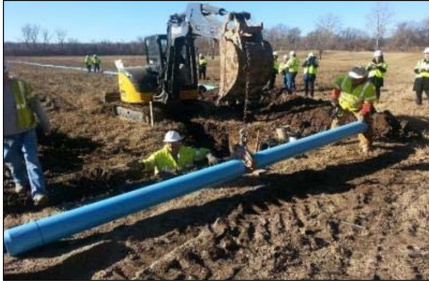
Figure 5.6 iPVC installation with manufacturer representatives on hand
