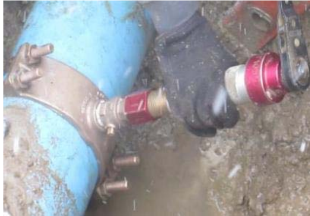
Figure 5.5 Tapping the iPVC pipe per AWWA guidelines
