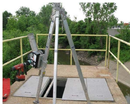
Figure 2 Confined Space Entry Staging
