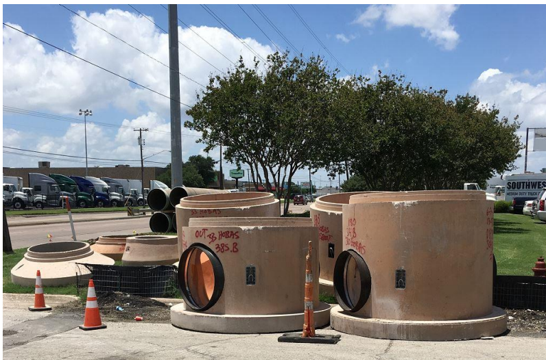
Figure 2.11 Pre-cast Antimicrobial Manholes
