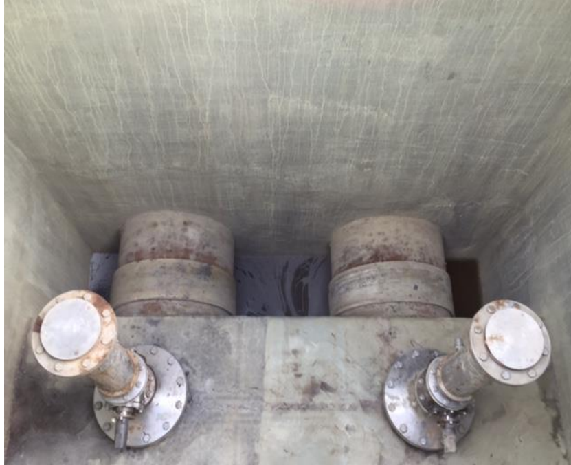
Figure 2.10 Air Release Valve Box 3 Years After Repair
