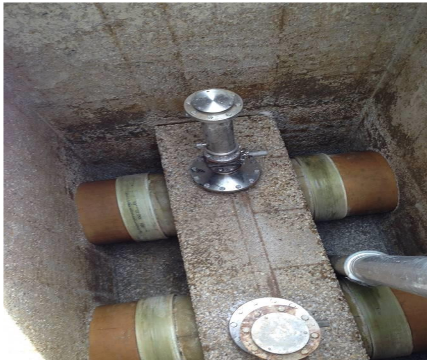
Figure 2.9 Walls of Concrete Valve Box after Pressure Washing
