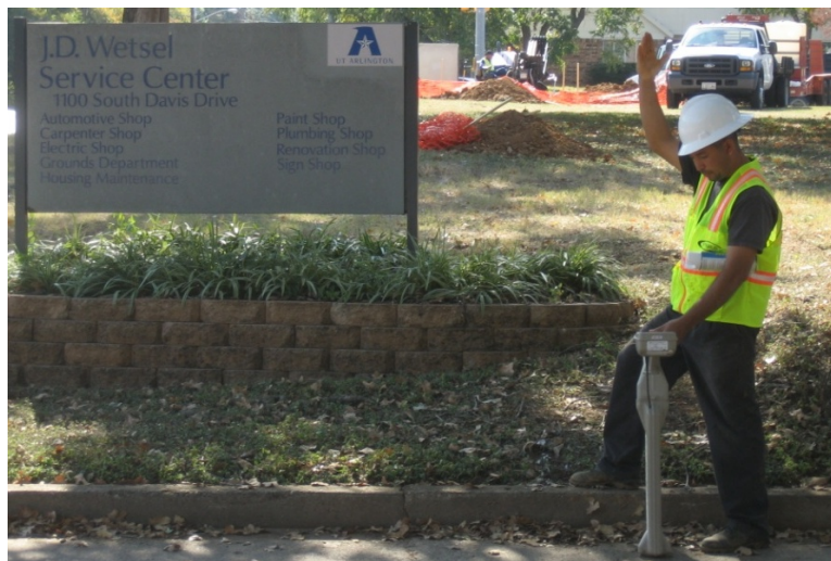
Figure 4-21 Drilling the First Run of Davis Drive Installation
