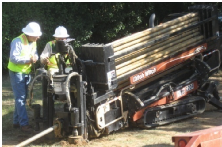
Figure 3-16 Ditch Witch JT2020 Used for Field Trials
