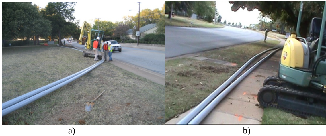
Figure 4-12 Pipe Location before Pulling a) East End, b) West End
