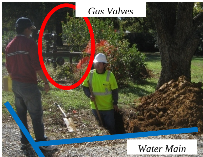
Figure 4-18 Potholing Water Main Line before Drilling
