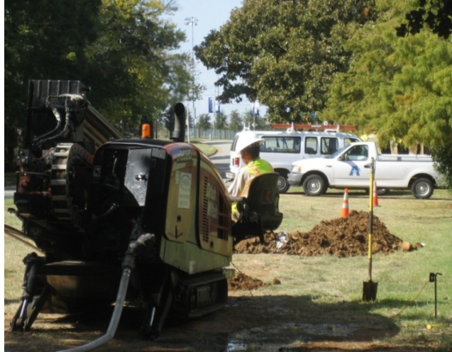
Figure 4-9 Drilling Pilot Bore Beneath Driveway (Second Run)
