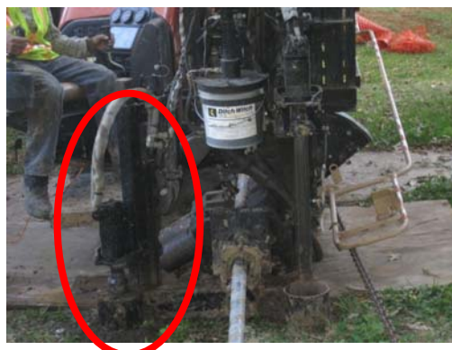
Figure 4-23 Breaking of mini-HDD's Right Anchor at Run 5
