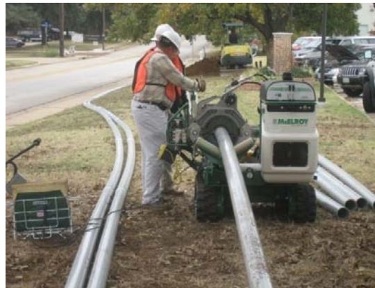
Figure 4-16 Pipes Being Added to Fused Line up to Desired Length
