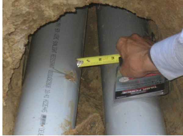
Figure 4-14 PVC conduits installed
