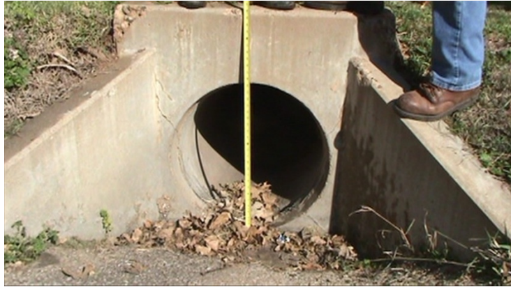
Figure 4-6 Culvert Inlet at Mitchell Street
