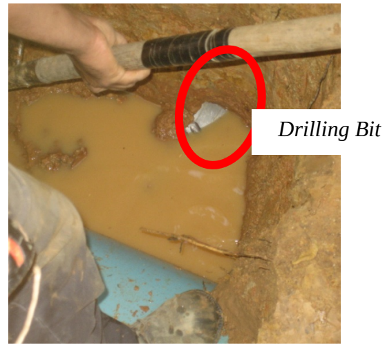
Figure 4-19 Drilling bit Close to Water Main Line
