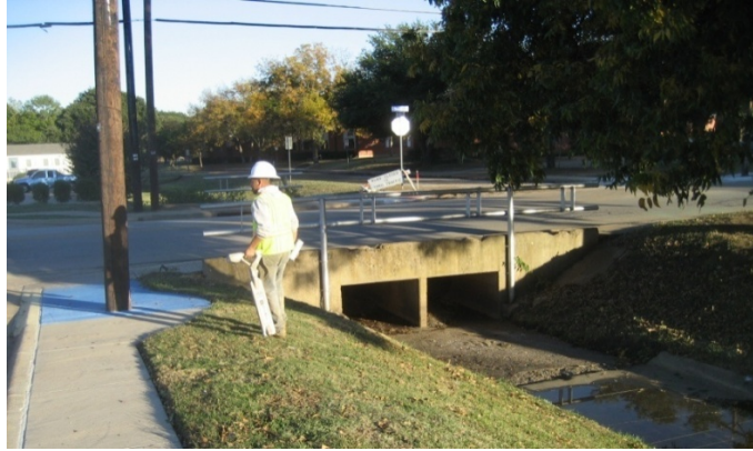
Figure 4-17 Twin Box Culvert at Davis Drive
